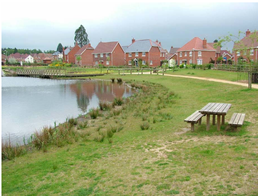
Example of SuDS in a new development, photograph by HR Wallingford
