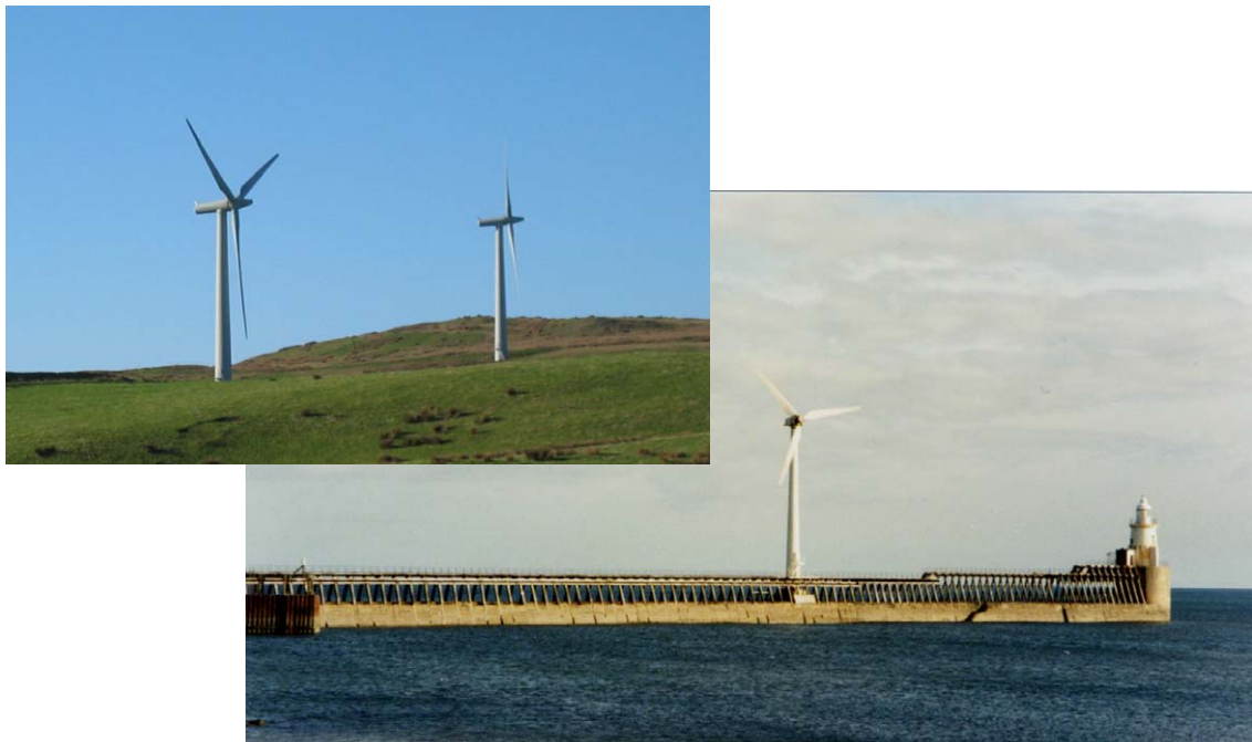
Images of wind turbines by HR Wallingford
